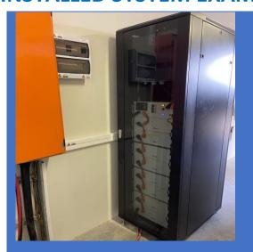
SIZE 50 KW 8 X 5.12 Deye 40KWh HV Lithium 24KWp Solar
