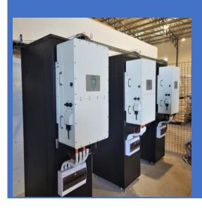
SIZE 150KW 36 X 5.12 Deye 184KWh HV Lithium 55KWp Solar
